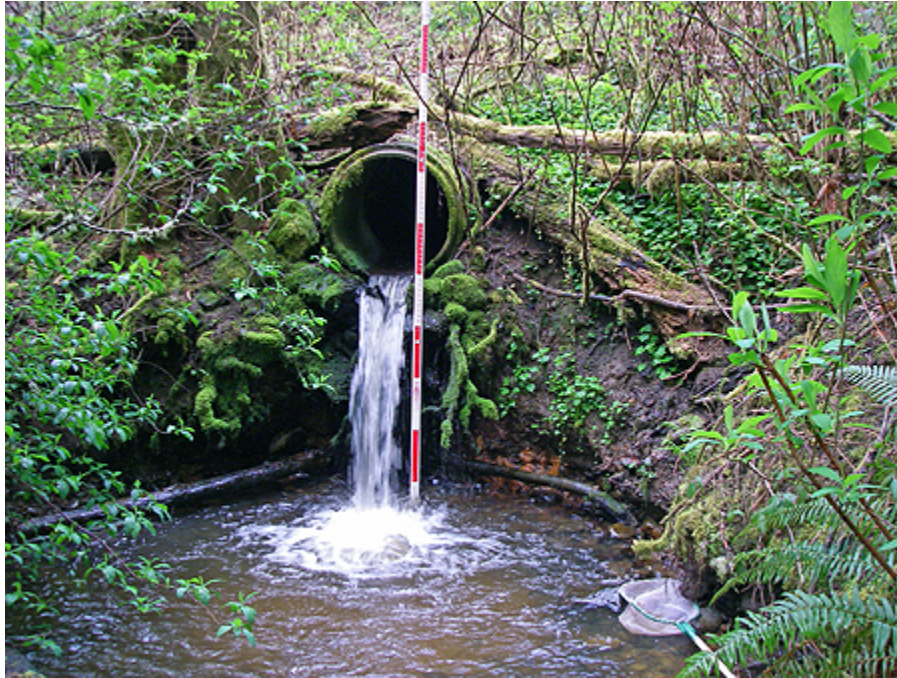
Photo 24 – Barrier culvert crossing of Leland Valley Road West on the 17.0078 tributary.
