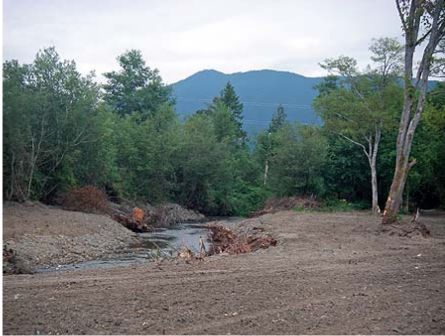
Photo 15 – Ongoing (August 2008) restoration of lower Little Quilcene River by HCSEG includes levee removal, construction of a meandering channel, supplementation with large woody debris, and eventual planting with native riparian vegetation.
