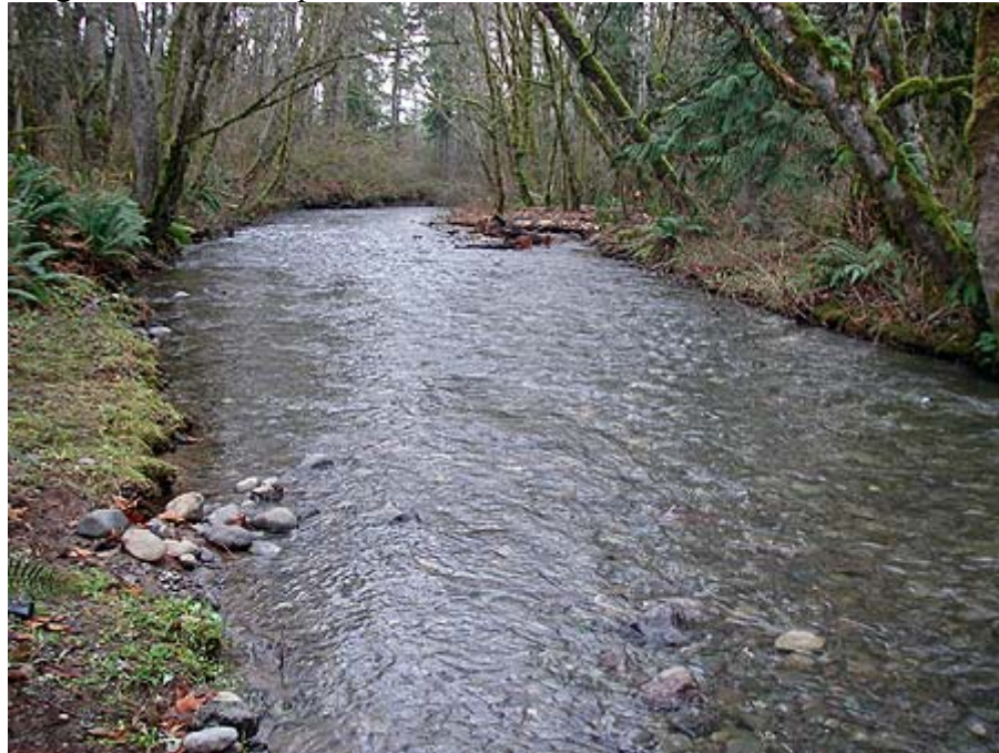
Photo 18 – View of the cobble diversion dam (remains are visible on left-bank) after seasonal high flows have flattened the dam and re-distributed channel substrates. Several logs are visible at the right-bank entrance to the “Wildwood Diversion Canal” downstream.
