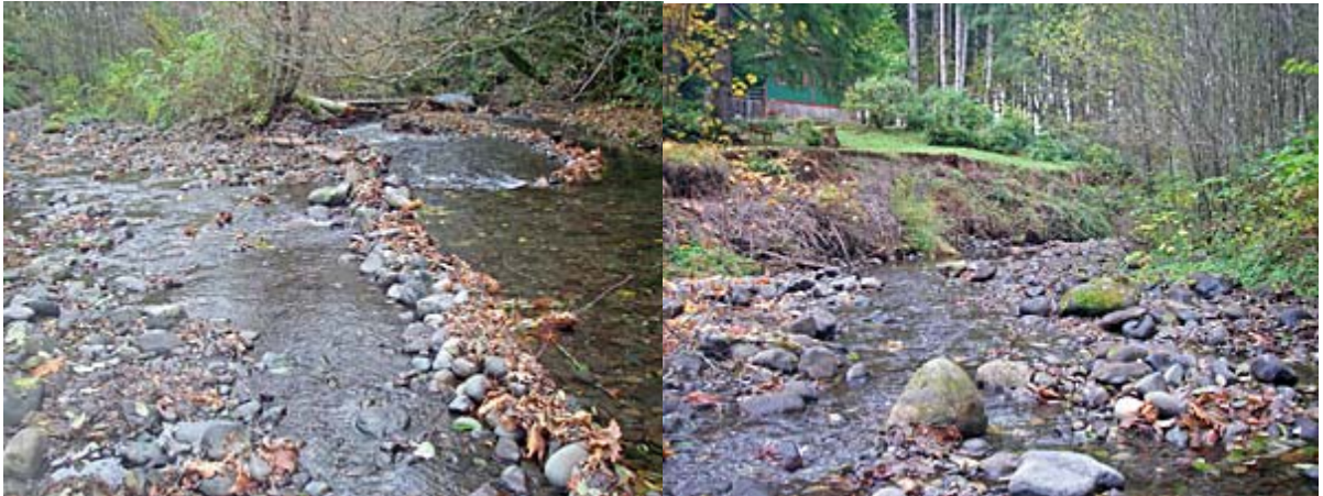
Photos 19-20 – Downstream view of another cobble diversion dam (left) near the upper extent of sub-reach 3b. “Push-up” dam diverts flow from an eroding left-bank bluff (right), but de-waters the downstream split channel.
