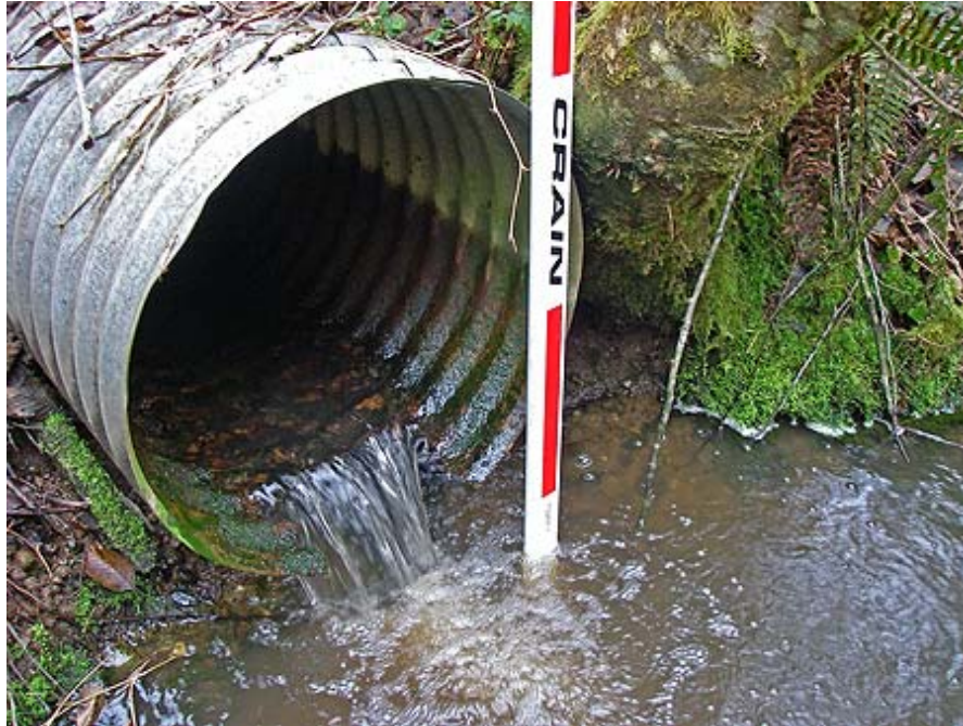
Photo 39 – Barrier culvert crossing of a decommissioned logging road along newly-mapped Type 3 habitat on a headwater reach of the 17.0017N tributary to Lake Leland.
