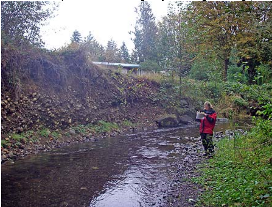
Photo 16 – Erosion of Little Quilcene River left channel bank (Reach 3, sub-reach 3a) at the site of a former bank stabilization project (note boulder riprap in background).
