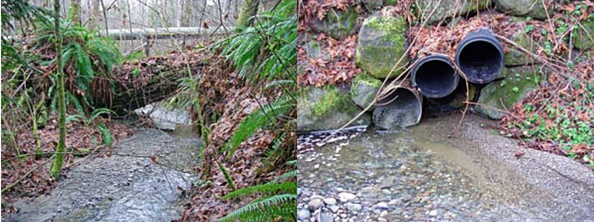
Photos 22-23 – A view of “Wildwood Creek” ~350 ft. upstream from the Little Quilcene River confluence (left), and ~50 ft. below a barrier culvert crossing of Big Leaf Lane (right). The “Wildwood Diversion Canal” crosses the Wildwood Creek ravine via a suspended aluminum pipe, and the culvert barrier disconnects several-thousand feet of potential mainstem and tributary anadromous habitat upstream from Big Leaf Lane.
