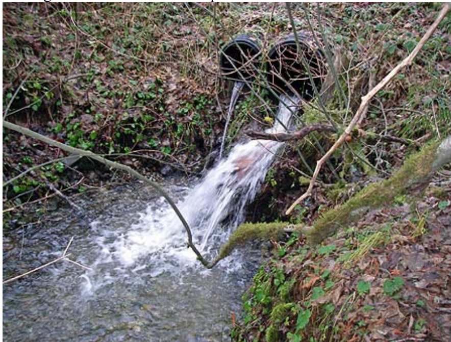
Photo 8 – Barrier culvert outlet at a private road crossing of a fish-bearing stream.
